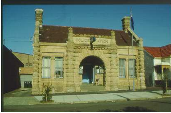
PLATE 4.3 Marrickville Police Station, significant public building. (A.P.1993).
