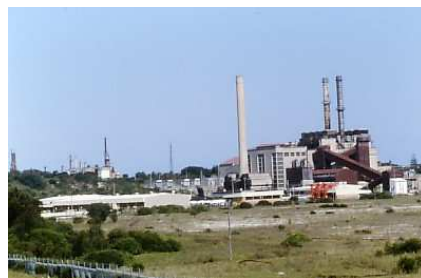
Bunnerong Power Station
